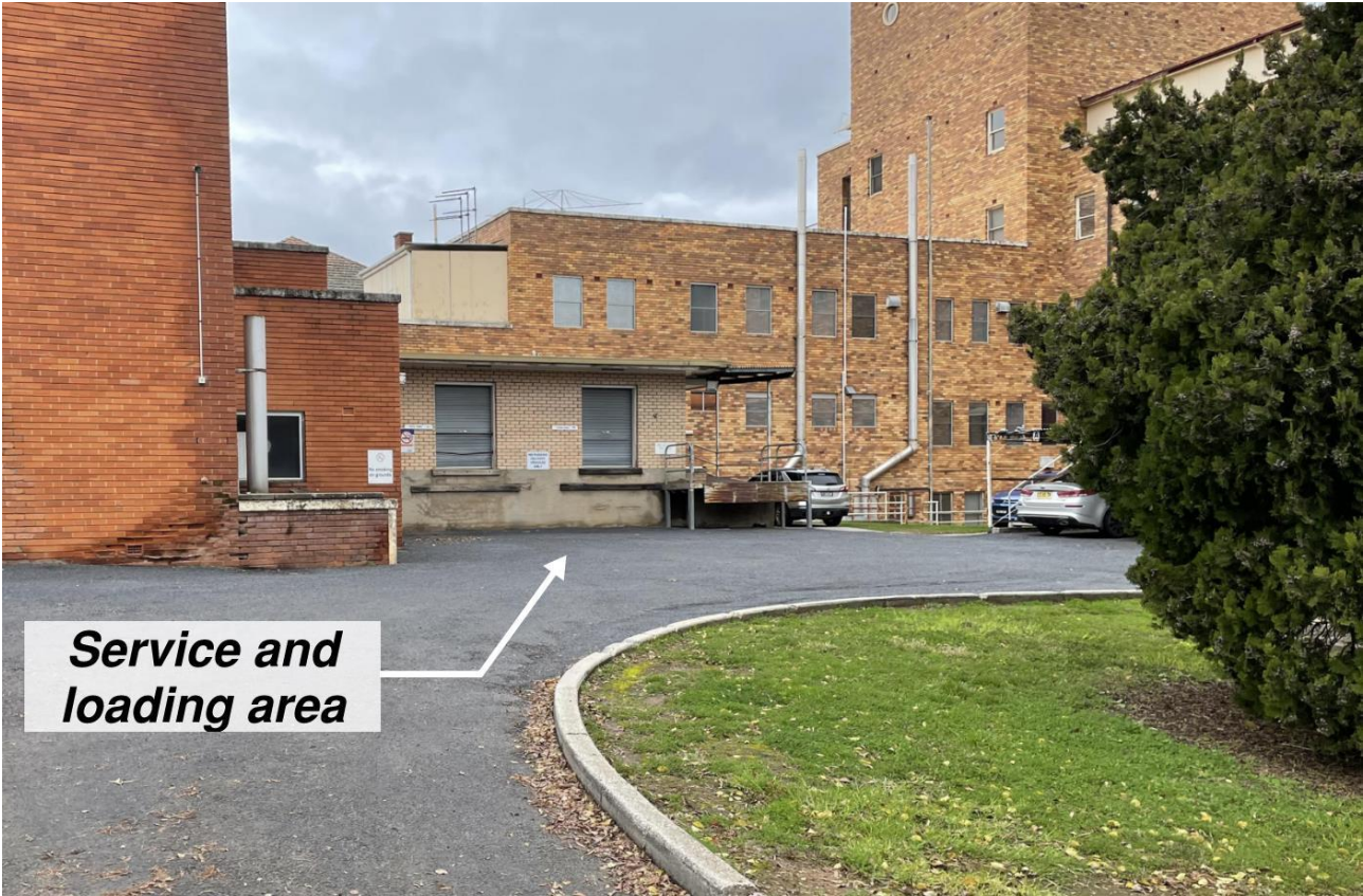
Figure 2.10: Existing Service and Loading Area
